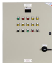
WATER MIST ELECTRIC MOTOR
